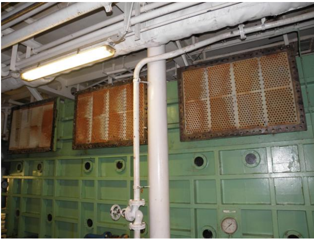
Evaporator Tube sheets
