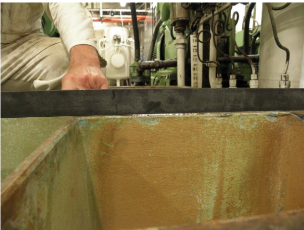
FDW reducing material space 2 a 3 mm
