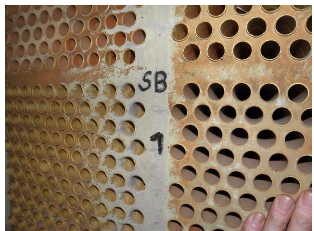
Space between ruler and tube sheet 5 a 6 mm
