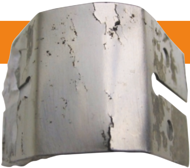
Element in stainless steel ceiling hook. The rust spots have been removed. Below rust spots, the material appears to be full of (micro) cracks. The sheet material has been cold-formed and is therefore full of internal stresses.
