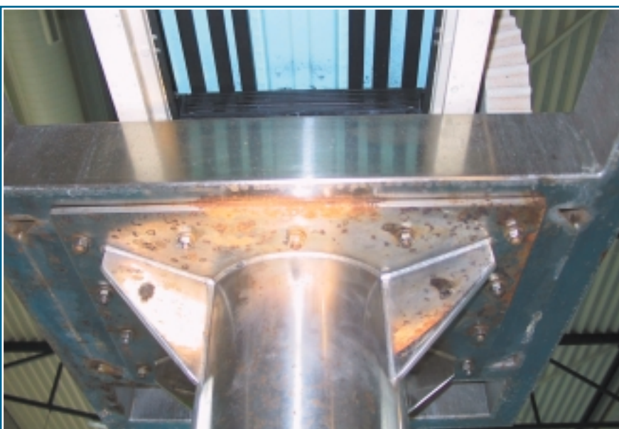
Rusted stainless steel AISI 316 construction, after six months' use.
